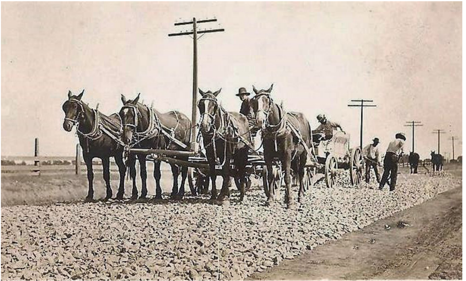
Highway construction in Galt circla 1914
